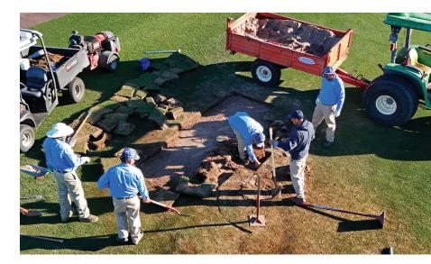
Underground leaks in lateral lines and mainlines are usually identified by wet areas at the surface. Repairs must be performed as soon as possible to ensure proper system function and minimize water waste.
