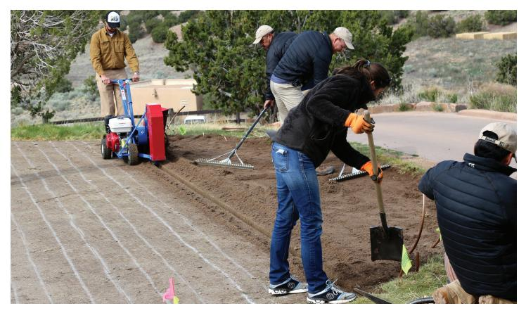
Installing SDI systems involves some disruption. Ideally, drip systems are installed into exposed soil where the surface can be easily smoothed out prior to grassing.
