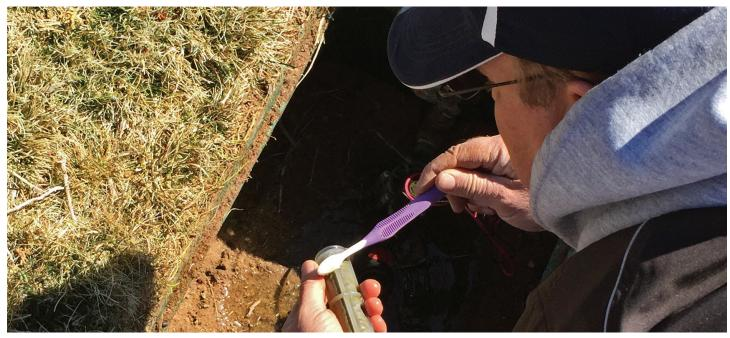
Checking and cleaning filters is part of the routine maintenance that is necessary to ensure SDI systems function properly. (Bernd Leinauer)
