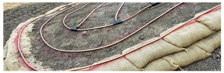
Irrigating the turf around bunkers is probably the most common current application for SDI on golf courses. It is a more effective and efficient way to water these difficult areas than overhead sprinklers or hand watering.
