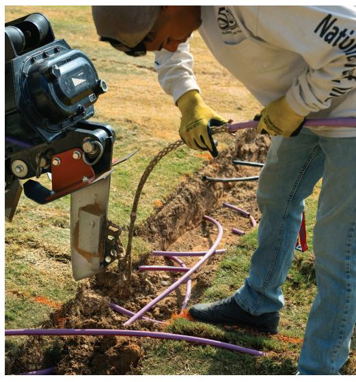
Installing SDI is more challenging and expensive over a given area of turf than installing overhead sprinklers. (USGA/Bill Hornstein)
