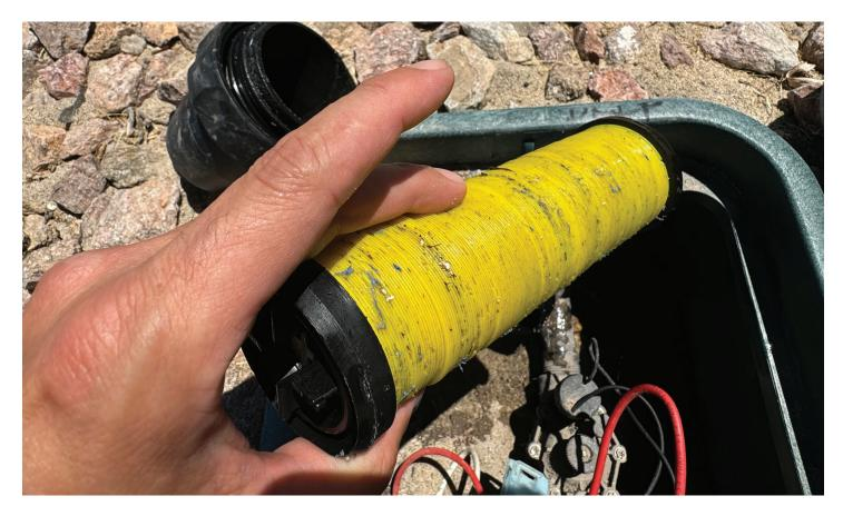
Disk filters are durable and require relatively little maintenance. They are typically used for smaller SDI systems and would be installed at the valve to the drip system.
