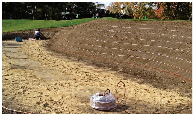
On steep slopes, like this bunker face, it is recommended to install driplines across the slope to limit the impact of gravity on flow through the pipes.
