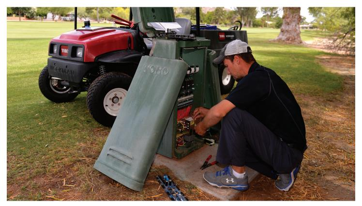
Satellites on the course should be inspected routinely for physical damage, wiring issues and the presence of pests or unwanted animals. (USGA/JD Cuban)
