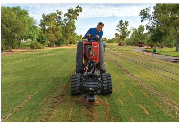
One method to install drip irrigation is by pulling the pipes. If pulling drip lines into existing turf, there will be surface disruption that needs to be addressed. (USGA/Bill Hornstein)
