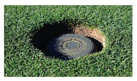
Turf growth, topdressing and sand splash from bunkers can elevate the surface around sprinkler heads. Low heads eventually need to be raised to ensure proper water distribution.
