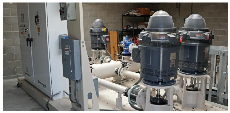
Visit the pump station regularly to check for any abnormal noises, operation when sprinklers aren't running, leaks and other issues.
