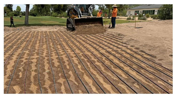
Once the SDI system is fully assembled and tested, cover the piping, grade the surface smoothly and install the turf.
