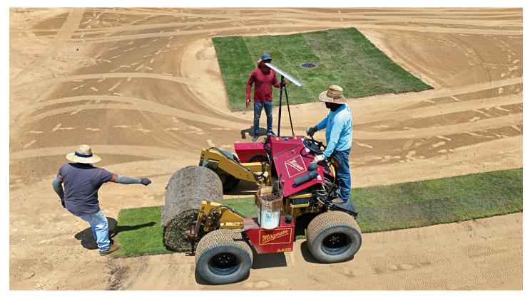
Sodding is more expensive than sprigging or seeding in terms of materials and cost to install, but quicker establishment with sod means less disruption to the golf calendar, better weed control and potentially a better finished product.
