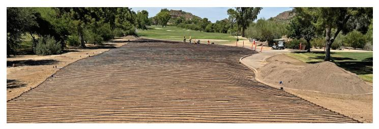
Removing turf and rootzone material prior to installing drip irrigation allows you to lay out, assemble, and test the entire system at the desired grade.
