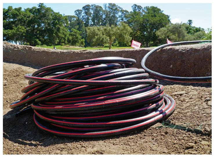
Drip tubing is commonly made of flexible polyethylene with an internal diameter of 0.5 inches.
