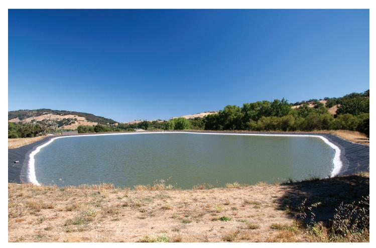
Most liners for golf course ponds today are made from plastic. While these liners are highly effective, they do require monitoring for damage, leaks or overtopping.
