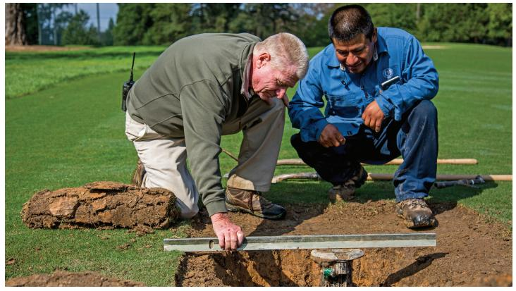
Keeping up with routine irrigation system maintenance isn't easy, but it's a great way to save water and improve playing conditions. Basic tasks like leveling heads and checking arcs can have a big impact. (USGA/Steve Boyle)
